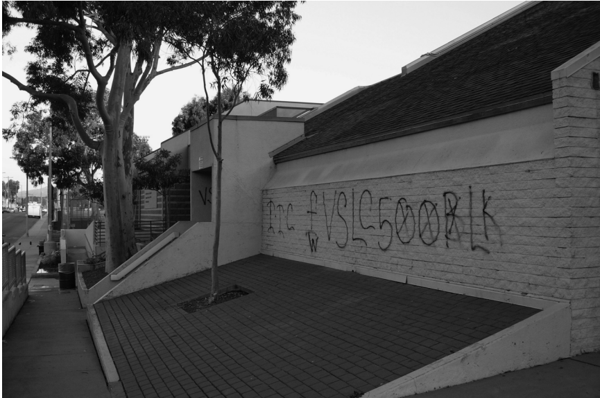
Figure 3 Photograph of the Oakwood Community Center with Venice Shoreline Crip Tag
